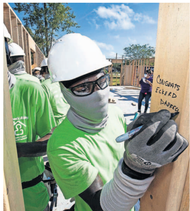
Darrell Wilkerson, with CareerSource Citrus Levy Marion and the Phoenix Rising YouthBuild program, writes a message on one of the studs used in a wall after about 30 people took part in the Raise The Wall event for the Jimarie Cruz-Sanchez home in Silver Spring Shore on Thursday.
