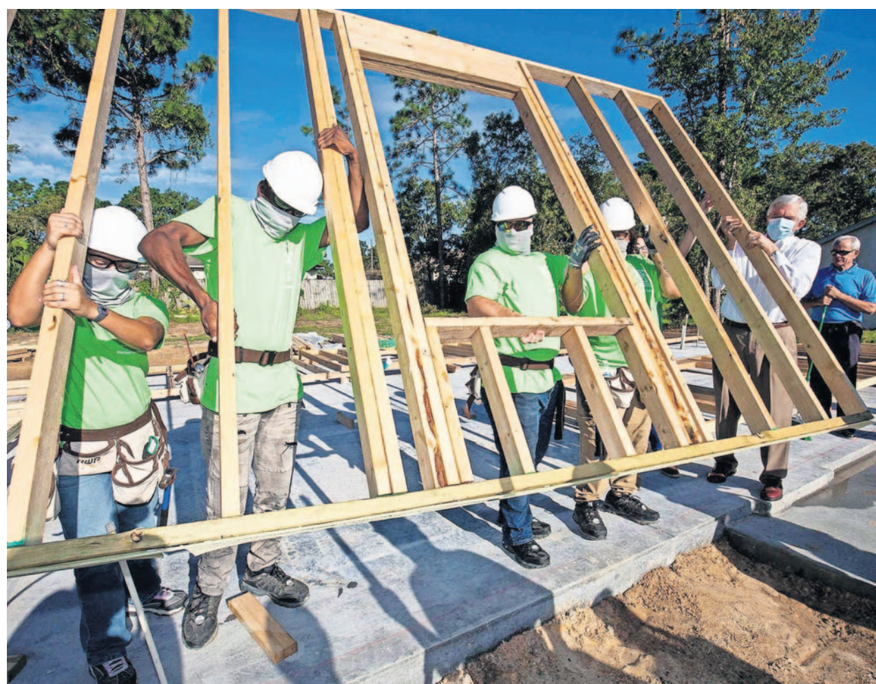
CareerSource Citrus Levy Marion and Phoenix Rising YouthBuild program members lift and place the first wall of the Jimarie Cruz-Sanchez home as about 30 people took part in the Habitat for Humanity Marion County Inc. Raise The Wall event in Silver Spring Shores Thursday. Over 250 homes have been built or rehabilitated locally since 1989 by Habitat for Humanity. [DOUG ENGLE PHOTOS/OCALA STAR BANNER]
