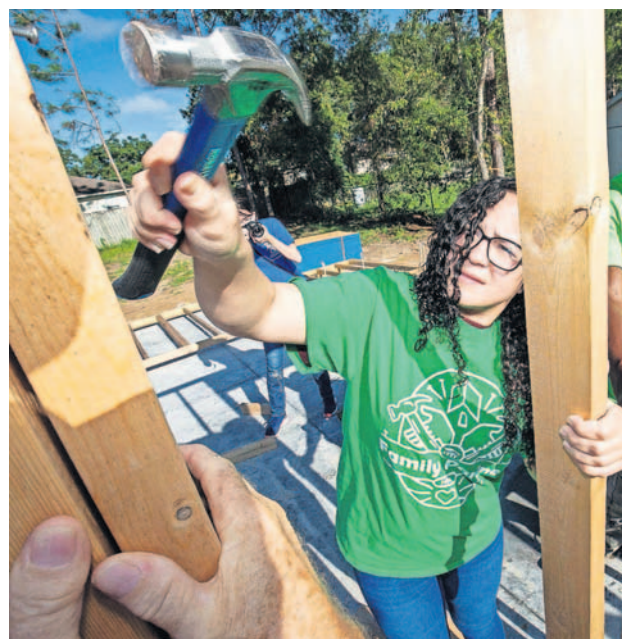
Jimarie Cruz-Sanchez hammers the first nail into her home as about 30 people took part in the Habitat for Humanity Marion County Inc. Raise The Wall event for the Cruz-Sanchez home in Silver Spring Shore on Thursday. The home, an 1,100-square-foot, three-bedroom and two-bath home will be built between 6 to 8 months. Jimarie will be moving in with her two sons when the home is complete.
