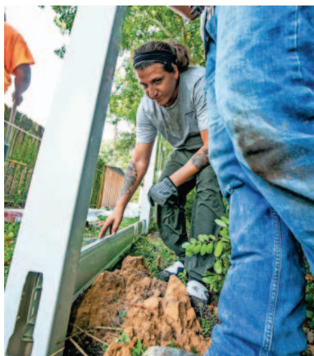
Nick Maglio, of Marion Fence, installs a vinyl fence Tuesday afternoon. Local businesses are struggling to find employees, with the top jobs available being cashiers, retail salespeople and fast food workers.
